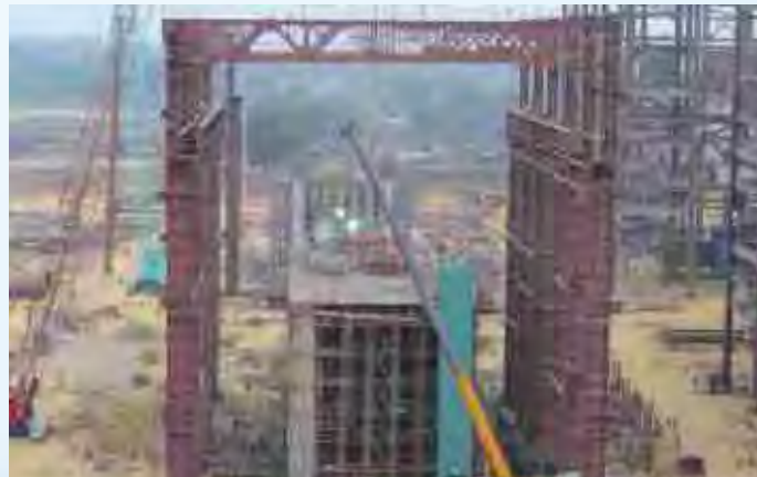
(In View: TG Building 3&4, TG Deck 3&4)
