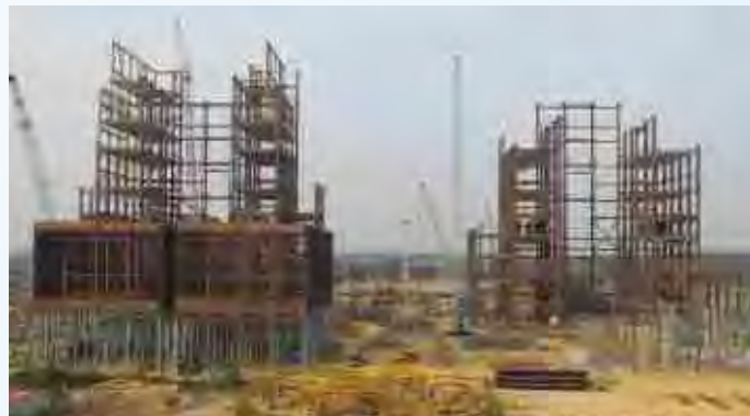
(In View: Boiler 3&4, ESP 3&4, Chimney)
